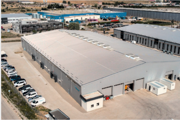
Company building from above
